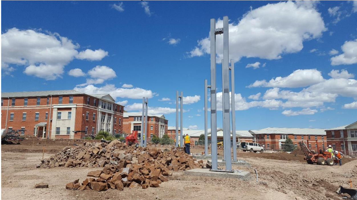
Beams for shade structure at Outdoor Amphitheater/Classroom (4/20/16)
